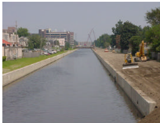
The Jefferson Parish Comprehensive Plan addresses issues relate to public facilities and infrastructure.
